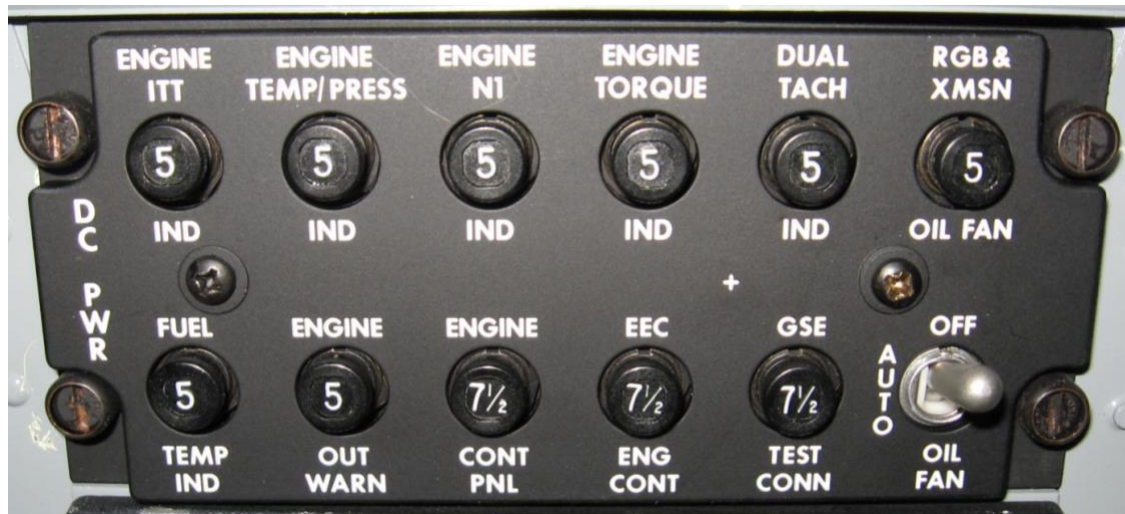
Figure 3-40 PT6 Circuit Breaker Panel
